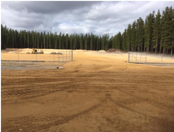
Figure 2a: Nangwarry-1 Well Site
